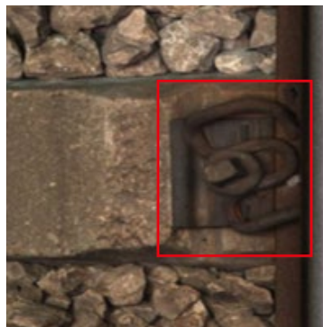
Displaced fastener
