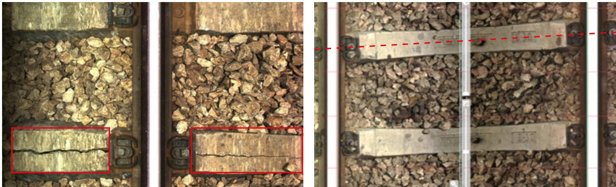
Recognition of sleeper and rail fixing elements defects: Sleeper cracks (left), Skewed sleeper (right)
